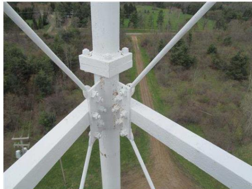
*Photograph 38: Old paint that was not cleaned off during last tower painting was visible on the inside gusset plate on the west leg in the first white color band from the bottom.
