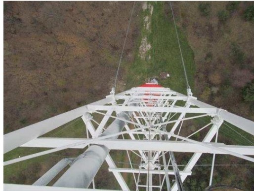
*Photograph 38: Old paint that was not cleaned off during last tower painting was visible on the inside gusset plate on the west leg in the first white color band from the bottom.
