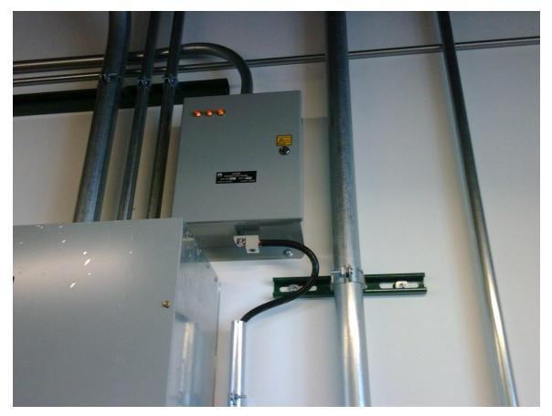
AC Power line protectors are a must – and they MUST be connected to your station reference ground.
